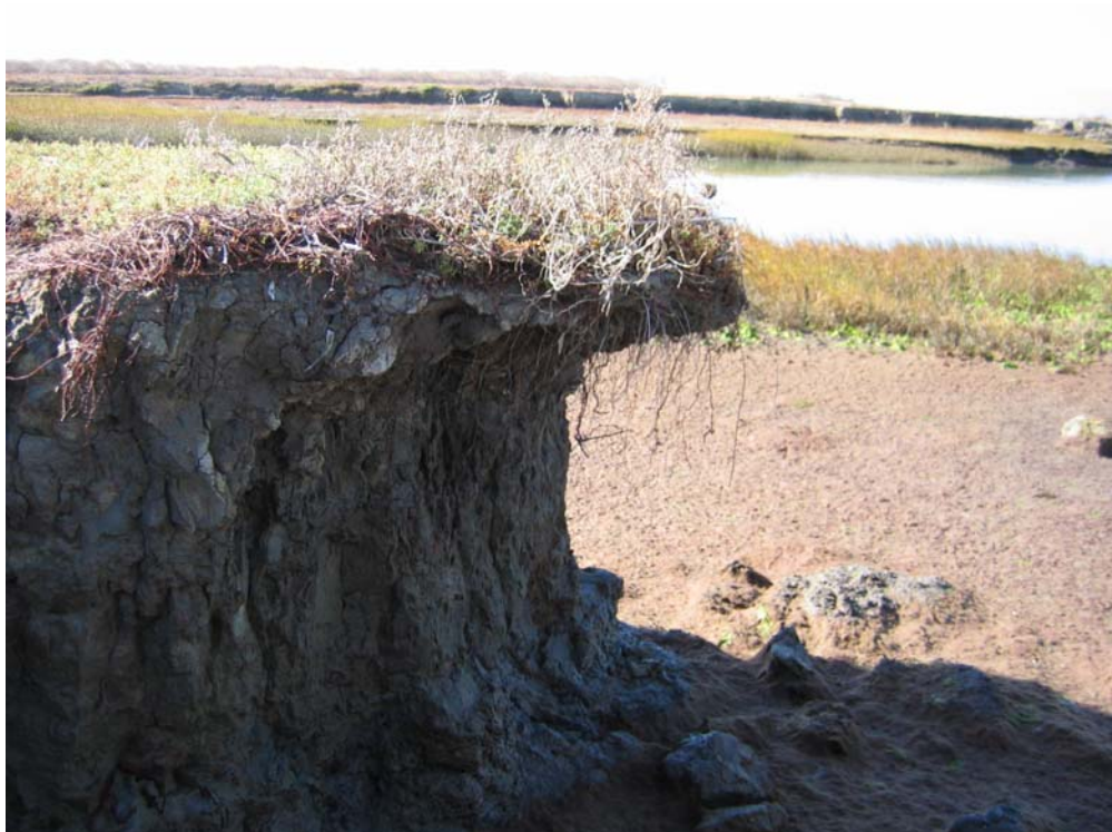
Photograph 8: Example of undercutting and severe erosion distress of levee slope (Pond BT1 Southwestern point)
